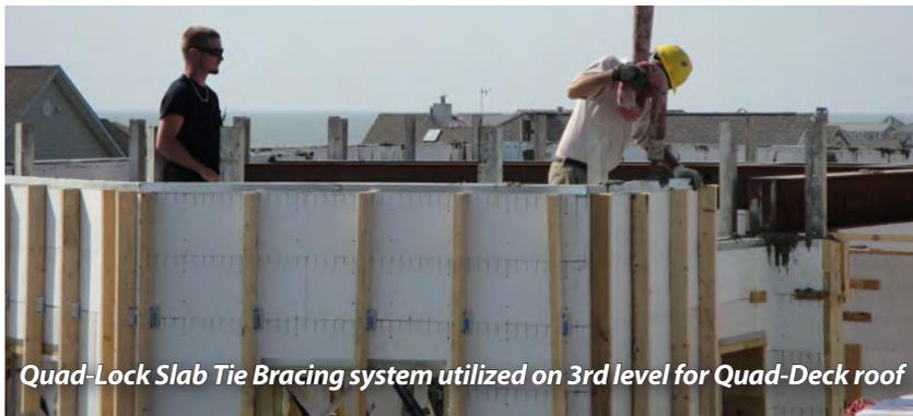
Quad-Lock Slab Tie Bracing system utilized on 3rd level for Quad-Deck roof
